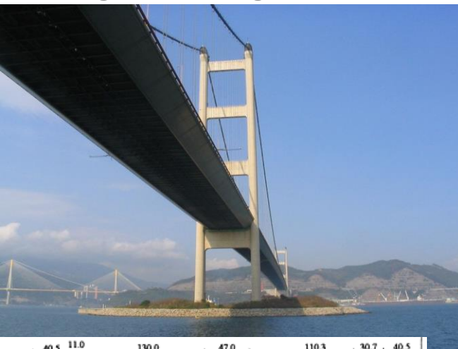
Tsing Ma Bridge (1377 m)
